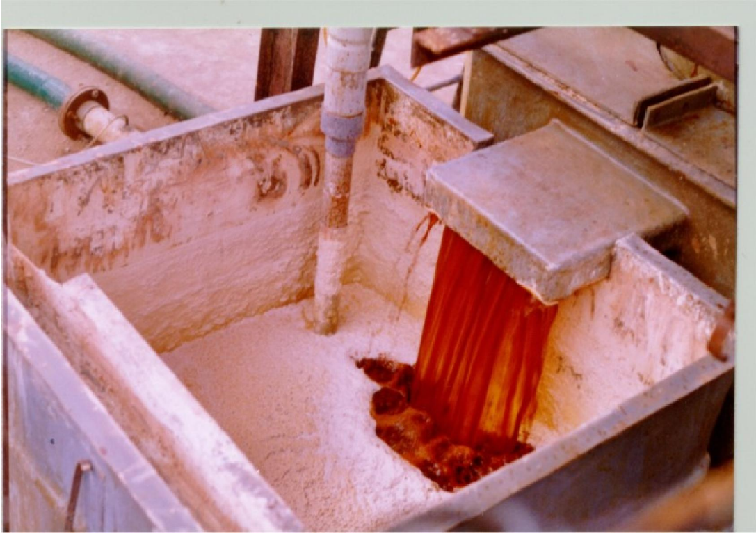
Picture of Scrubbing Solution & Precipitated Sulphur used in ISET Process
